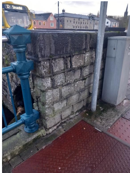
Plate 7 –The modified wing walls (southern side) are comprised of coursed limestone blocks, with heavy strap pointing
