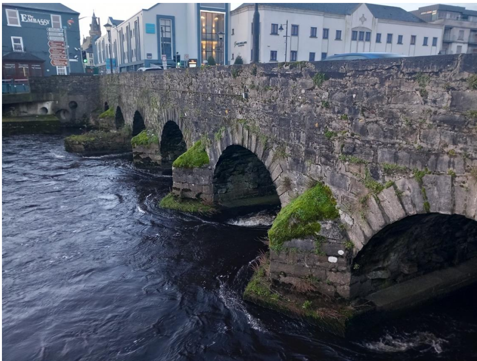
Plate 2– Dressed limestone voussoirs on the upstream elevation
