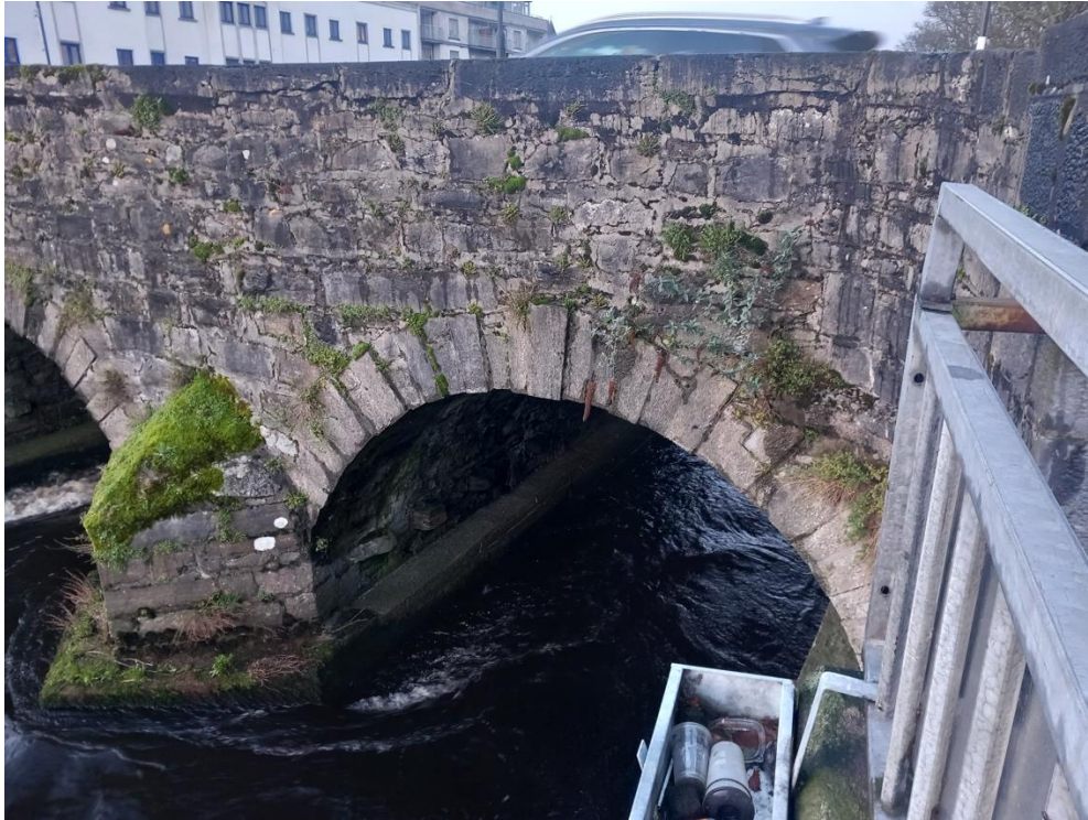
Plate 3 – Detail of dressed limestone voussoirs with keystone. Vegetation is apparent on the spandrel walls and cutwaters
