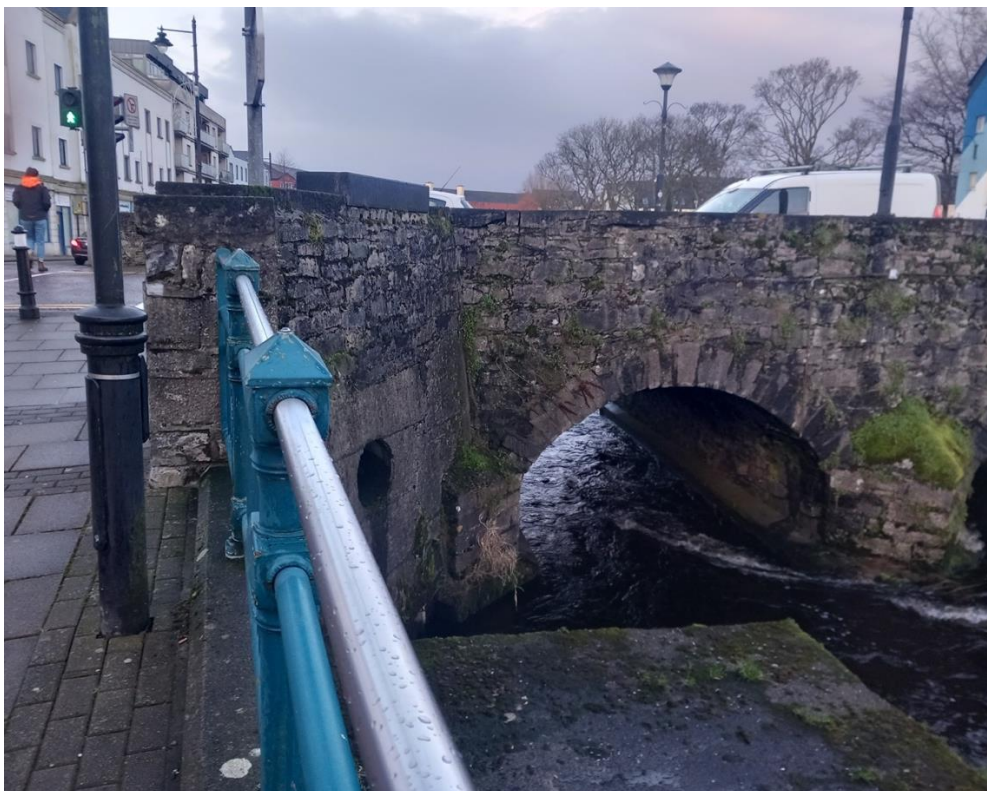
Plate 4 –The southernmost arch has been partially infilled and the parapet walls modified adjacent the southern bank
