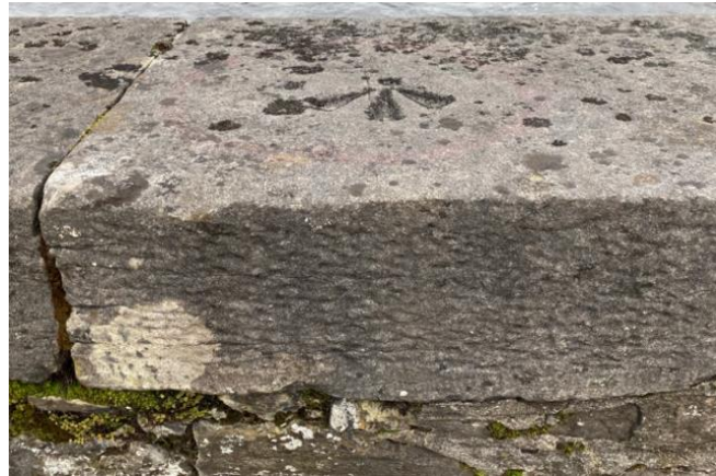
Figure 12 – Benchmark cut into capstone of eastern parapet
