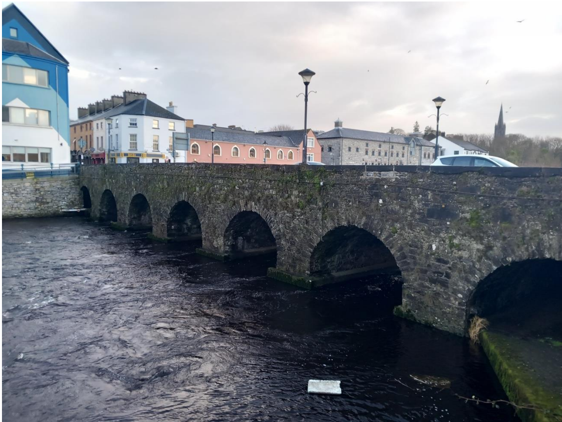
Figure 13 – Western elevation of Markievicz Bridge. The southernmost arch have been partially infilled, and the concrete base is exposed at low tide
