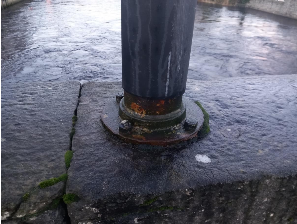
Plate 8 –Detail of base of lamp standards bolt fixed to limestone parapet walls
