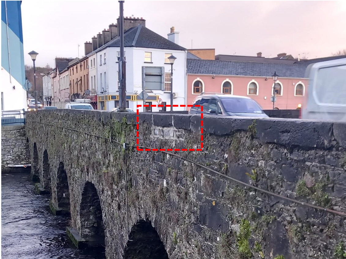
Figure 14 –Inappropriate mortar and repointing style, as evidenced in the highlighted area can injure the appearance of the bridge and where cementitious mortars are used, they can cause physical damage to the adjacent limestone
